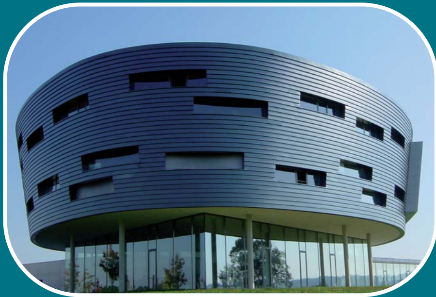
Cancom HQ, Jettingen, D, Granex Black Colour Tex
